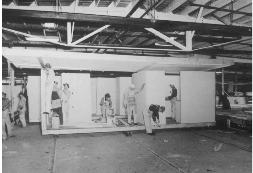
Image #20: TVA Indoor Prefabrication Plant (TVA Archive, National Archives Building, Atlanta, GA.)
