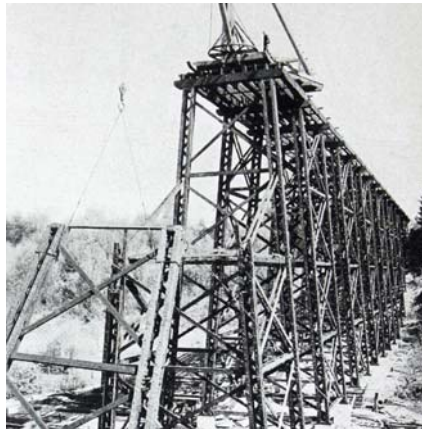
Pre-framed and treated composite trestle bridge: Port Angeles, WA
