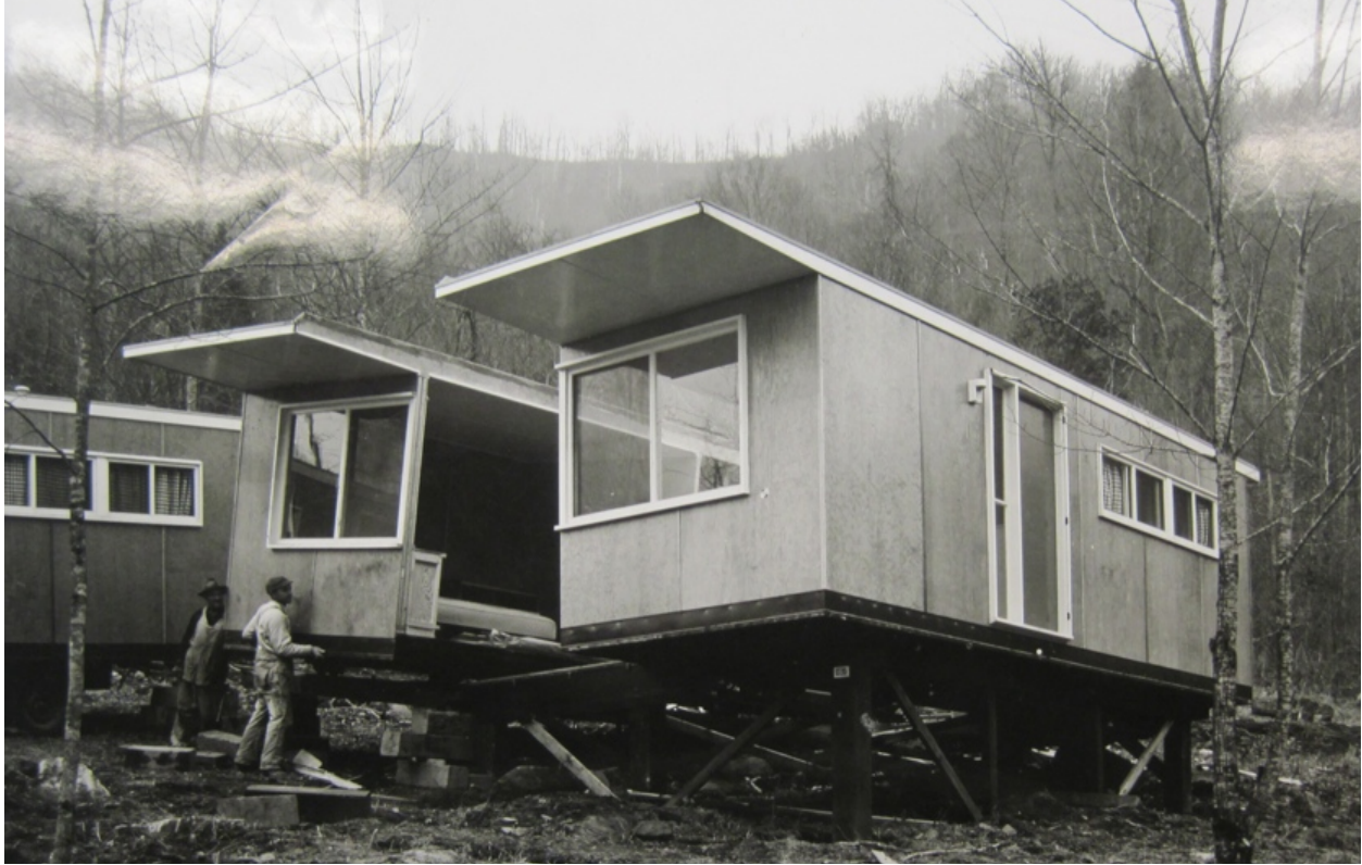
Image #15: Constructing a TVA "Truckable" House (TVA Archive, National Archives Building, Atlanta, GA.)
