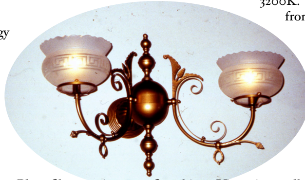
Glass fibre optics retrofitted into Victorian wall sconce on 100' atrium. This replicates the color and light level of the original gas fixture
