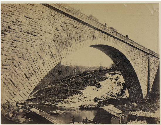
Union Arch / Washington Aqueduct
