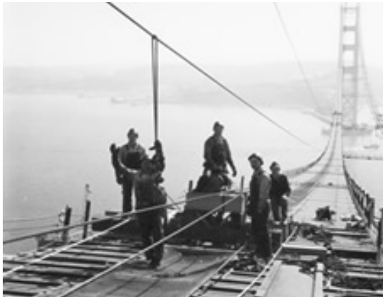
Main Cable Spinning
